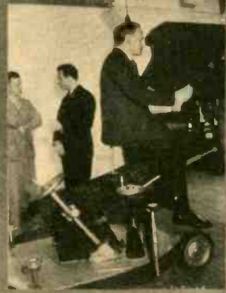
Above—One of the CBS television experts is here seen trying out one of the image pick-up cameras, which is provided with a crane and seat so that the operator can swing around while televising the players in the studio. Frequently two cameras are used, one for close-ups, and one for long shots.
