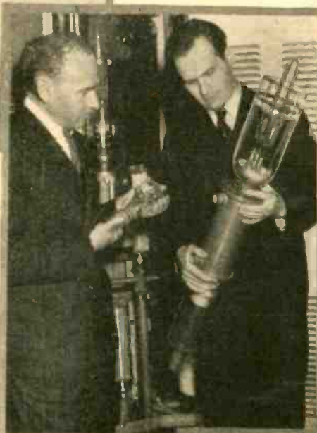
Right—Tubes for Television. Gilbert Seldas (left, television program director, and D. Peter Goldmark, chief television engineer, inspect the largest and smallest water-cooled tubes used in the new CBS television transmitter. The large power tube has 15,000 watts peak output and is three feet long.
