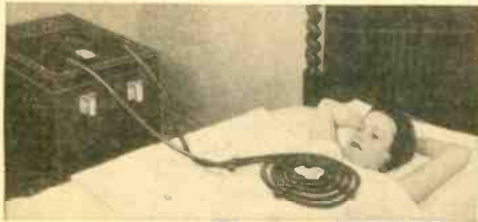
Here is a different technique in applying the high frequency field, the currents circulating in the coil producing a field which passes through the body.
